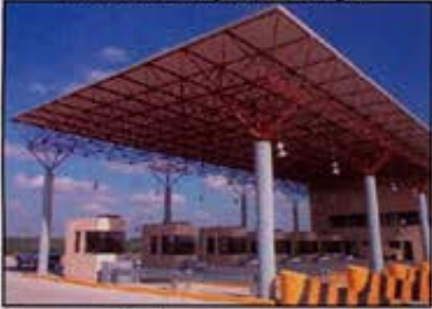
Toll station canopy
