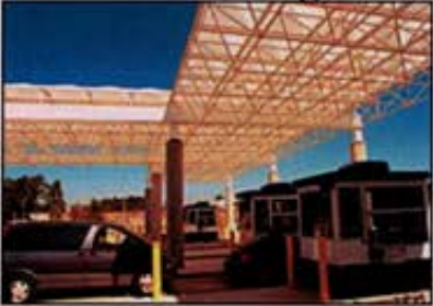
Air port parking exit
