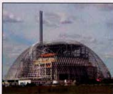
Marchwood dome under construction
