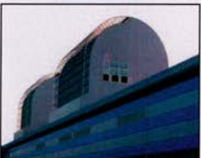
Galvak steel coil painting facility
