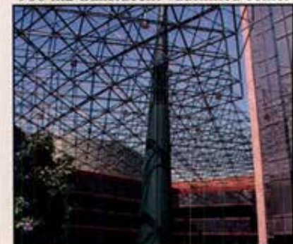
Office complex central plaza
