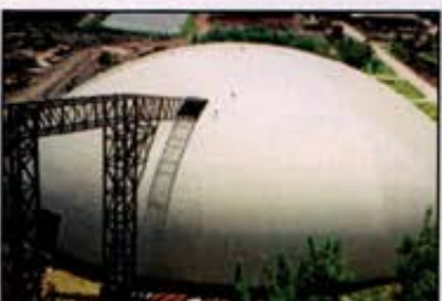
125 m ring pile dome , Thailand
