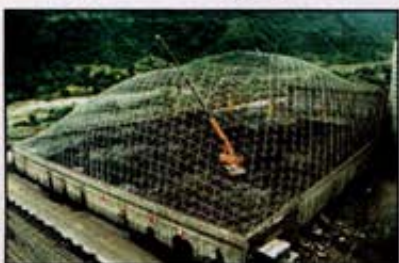
Construction of dome on 35,000 ton
