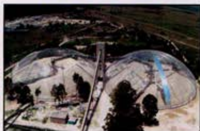
2 x 113 m limestone storage domes under construction , south africa
